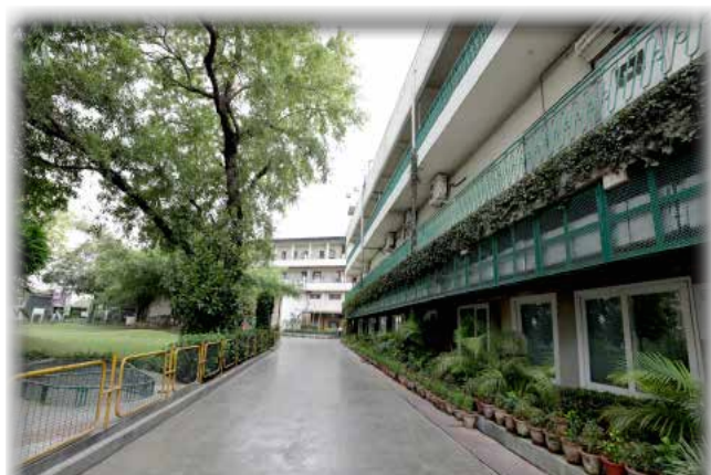
Administrative Block at Factory- MIL Hapur
