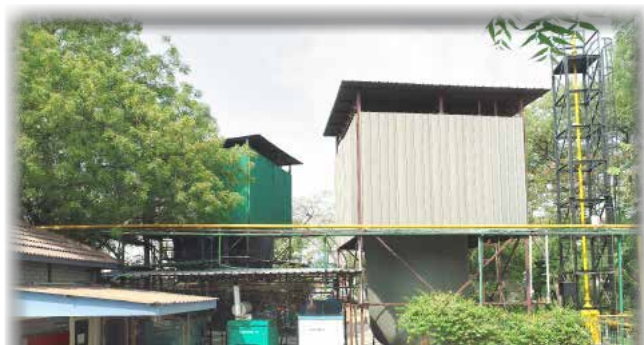
Bio Gas plant in MIL unit-1
