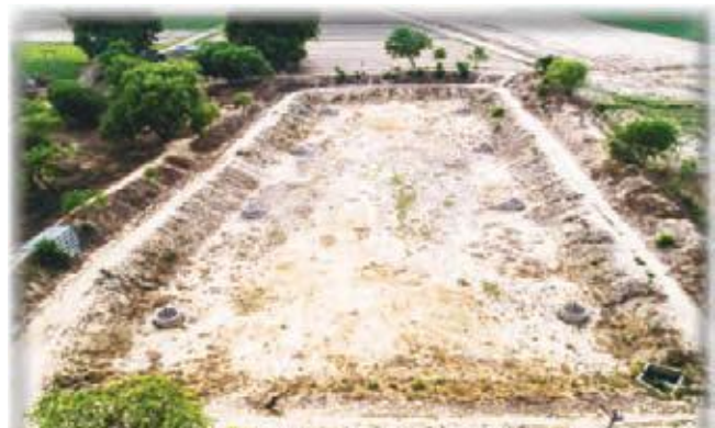
Newly constructed pond for water recharge at MIL-2 unit of Hapur
