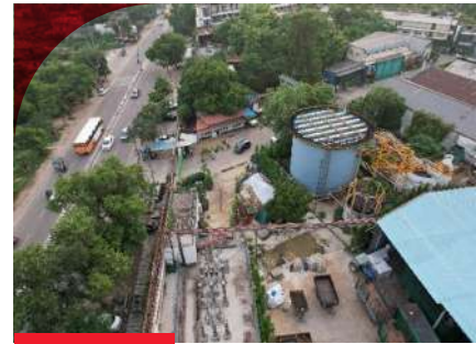
Ariel view of Anaerobic Digester
