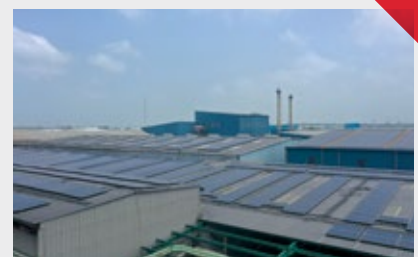
Rooftop Solar, MIL Rohad
