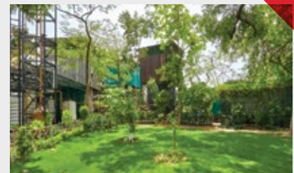
Bio compost and Biogas unit, Hapur
